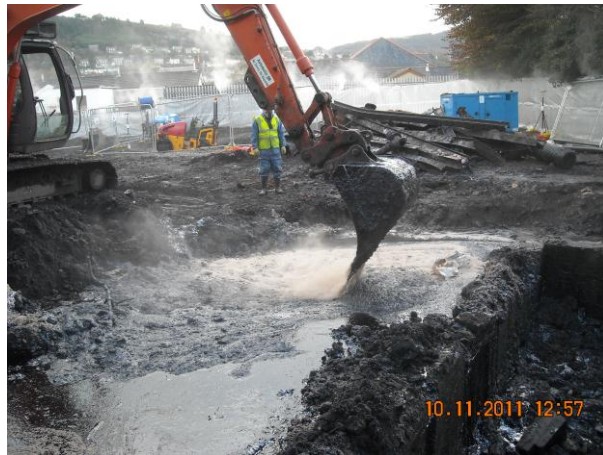
Figure 2. Remediation at Briton Ferry Gas Works
